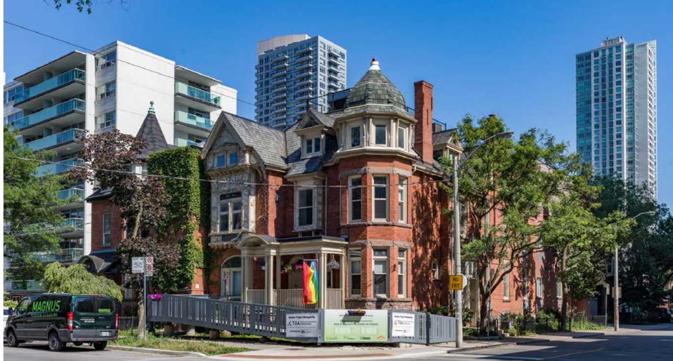
A wheelchair ramp offers accessibility to the Fife House, a historic renovation near downtown Toronto that provides services to people with HIV/AIDS who are also experiencing homelessness.
